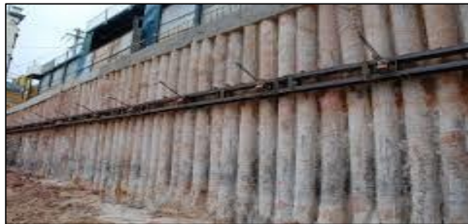
Figure 1: A contiguous pile wall sample
