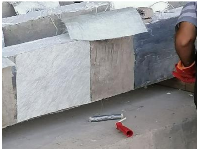
Figure 5: The installation process of GFRP sheets
