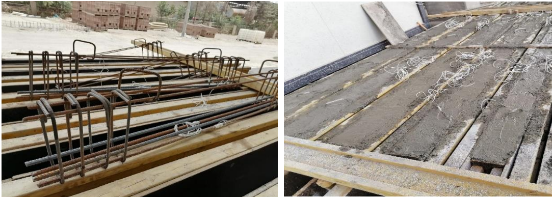
Figure 4: Steel reinforcement case of the beam specimens
