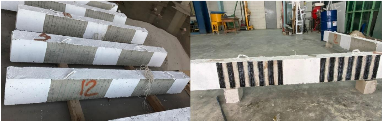
Figure 4: Preparation of concrete beam surface and applying CFRP strips
