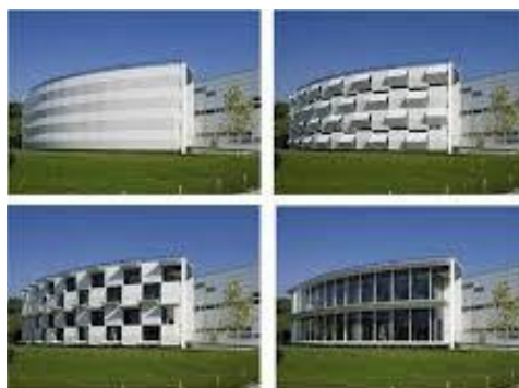
Figure 12: Kiefer showroom" building, Austria,Graze
