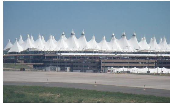
Figure 2: The DIA Terminal's remarkable roof design [6]
