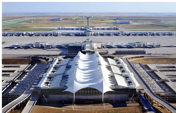
Figure 11: View of the fabric roof of DIA [26]
